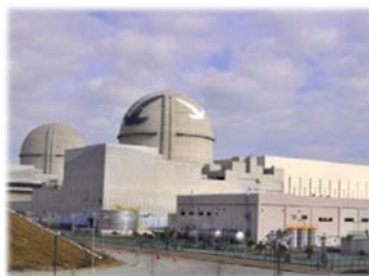
Nuclear Power Plant (S.Korea)
