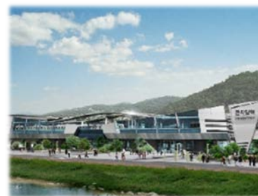
Subway Station (S.Korea)
